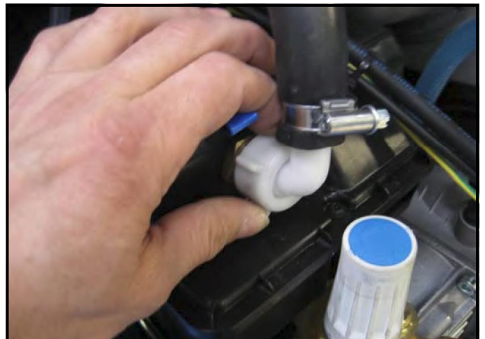
Fig.F.91: Water break tank.
